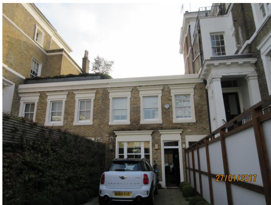
View from street (top) and closer front elevation (bottom).
