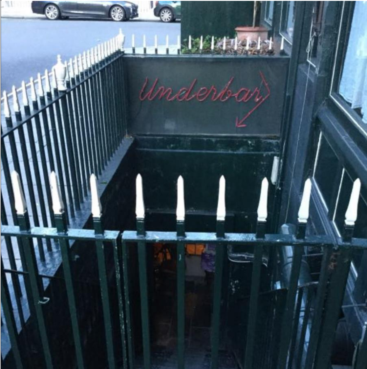
Existing external entrance to basement (and proposed bakery)
